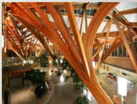
Carlo Fidani Regional Cancer Centre, Mississauga, ON
